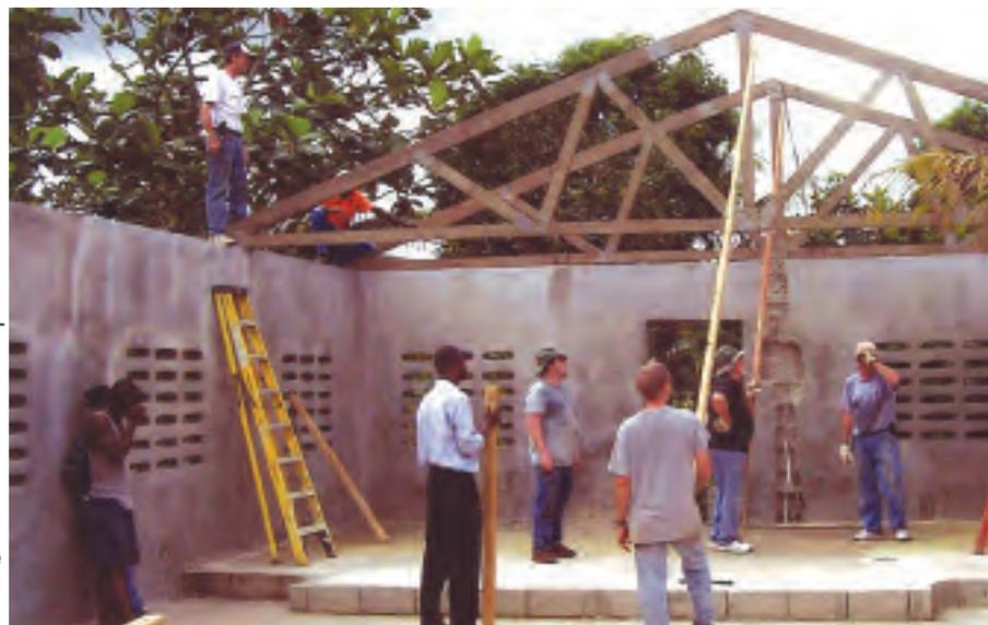
The Illinois church team at Plain de Nord church site, hoisting roof trusses into place.
