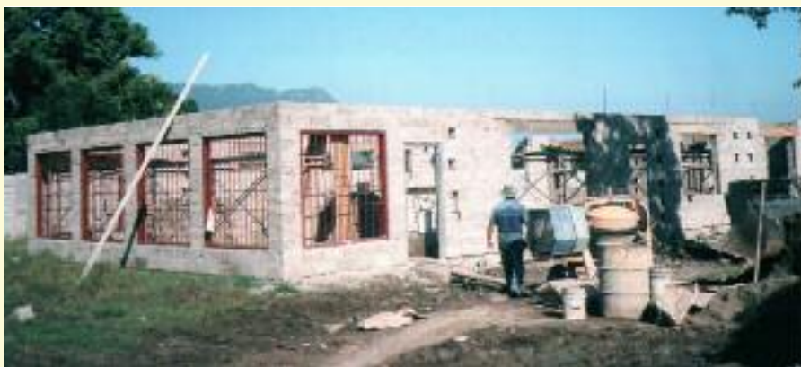
Emmaus Biblical Seminary under construction.
