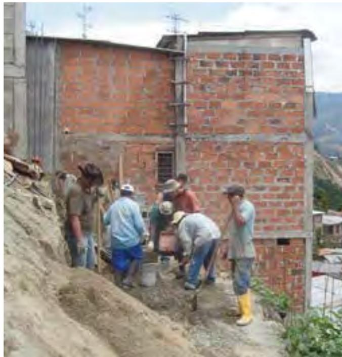
**Making concrete at the Olaya church project to build retaining wall at edge of 20' drop-off.**
