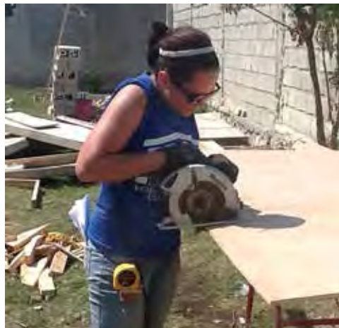
Briana learning a skill at construction site.
