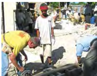
Tulsa team preparing forms for cement.
