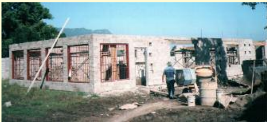
Emmaus Biblical Seminary under construction.
