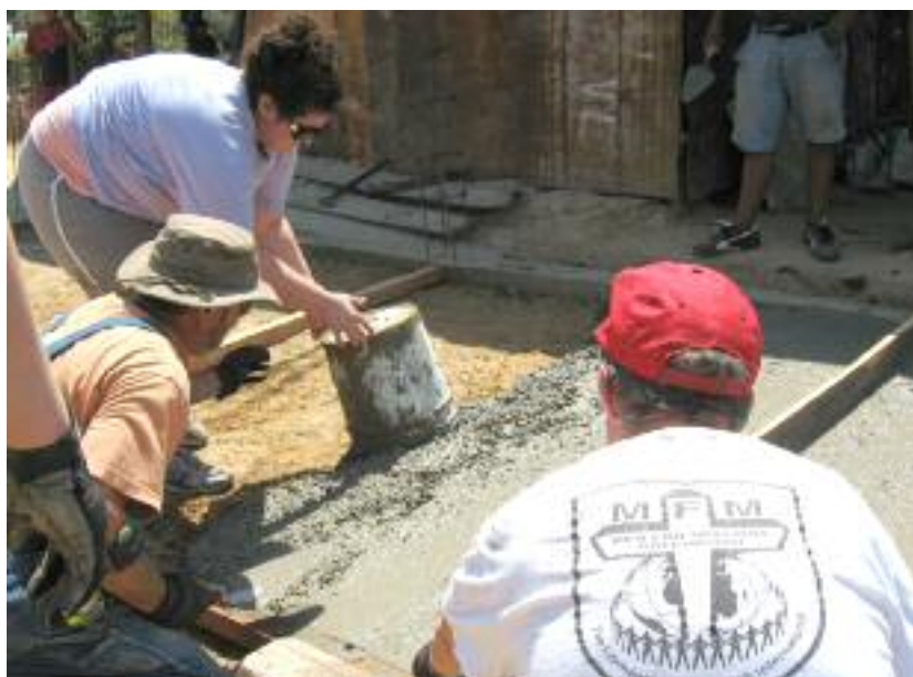
MFMI work team pouring concrete.
